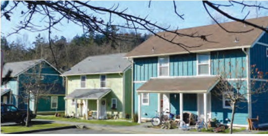
The six-month, $900,000 renovation of the Lavender Hollow apartments included new siding, roofing, windows, ventilation, and landscaping. The project was funded by a grant from the Washington State Housing Trust Fund.
