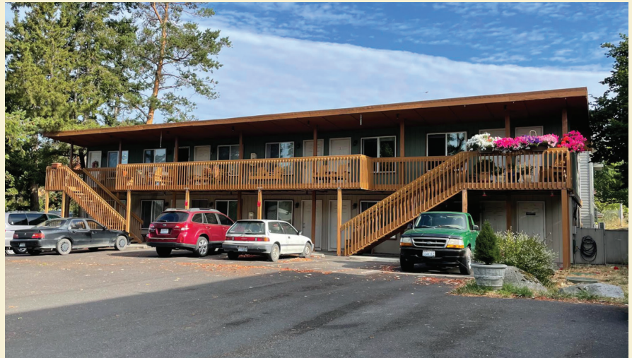
Northern Heights apartments in Eastsound Village.
