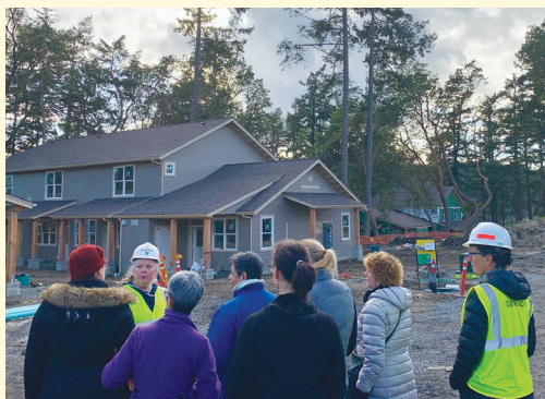
This spring, OPAL led a tour of the April's Grove site for the Orcas Community Resource Center (OCRC) to check out construction. The OCRC is an important resource helping some clients apply for April's Grove.
