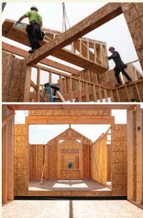
The walls are going up! Construction of OPAL's five new Lydia Lane homes is well underway at West Coast Homes in Lynden.
