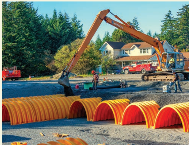
What began as a vision is becoming a neighborhood! Work continues at Pea Patch, bringing Orcas Island one step closer to 20 new affordable rental homes.
