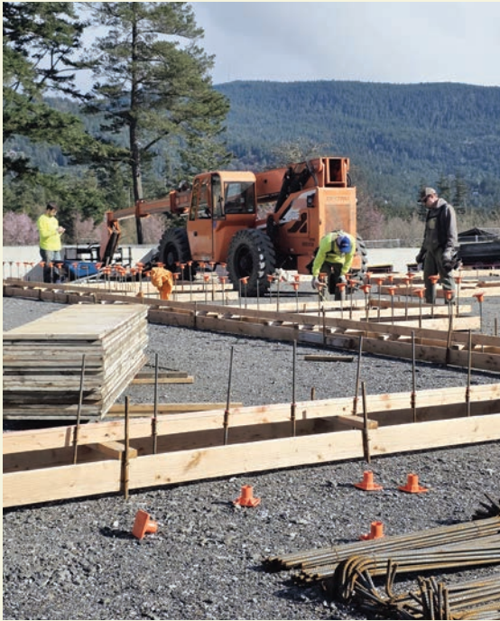
Laying the groundwork for new beginnings at Kidder Way.
